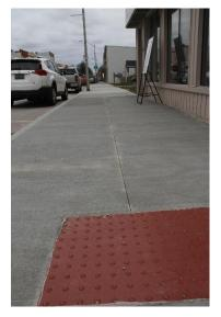
Downtown Norwich sidewalk along the south side of Main Street from Pitcher Street around the corner at Stover street to Front Street. Sidewalk was rebuilt and wherever possible the sidewalk was the sloped to the business entrance to allow for accessible entrance instead of a step. Tactile strips were installed at intersections.
