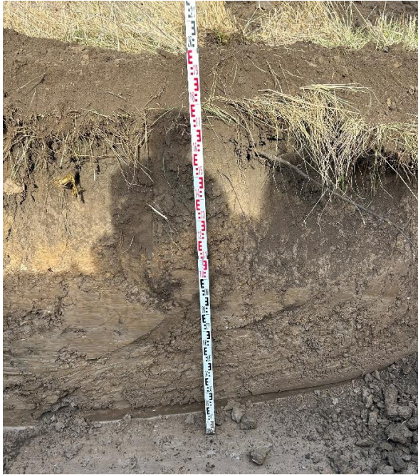
Figure 3 – (Left) Soil conditions observed at TP#3
