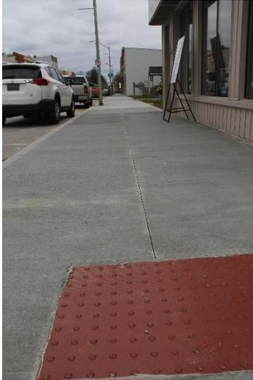
Downtown Norwich sidewalk along the south side of Main Street from Pitcher Street around the corner at Stover street to Front Street. Sidewalk was rebuilt and wherever possible the sidewalk was sloped to the business entrance to allow for accessible entrance instead of a step. Tactile strips were installed at intersections.
